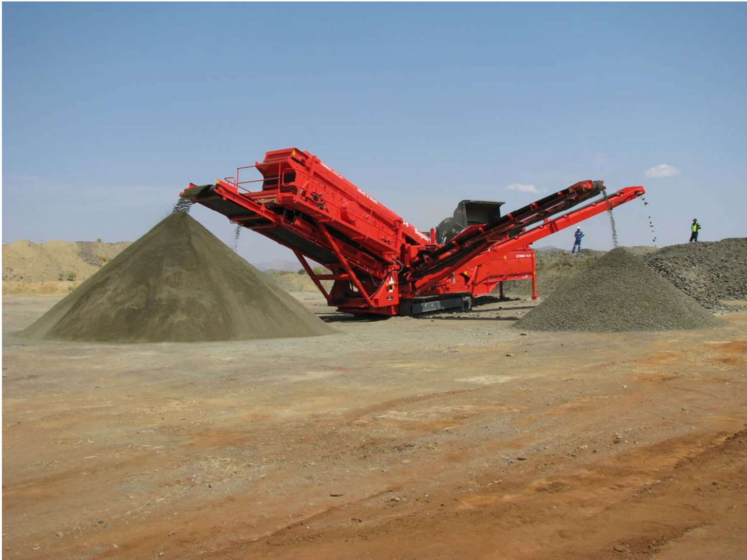
Stellite Chrome Project - Crushing and Screening Plant
